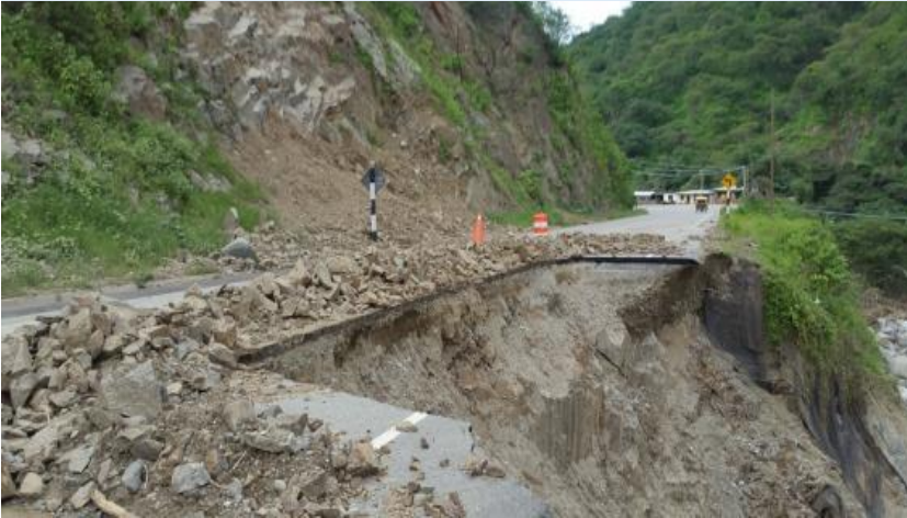
Km. 17+480 al Km 17+730 – Tramo 4
