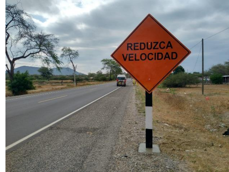
Km197+600 – KM 197+680 - Tramo 5
