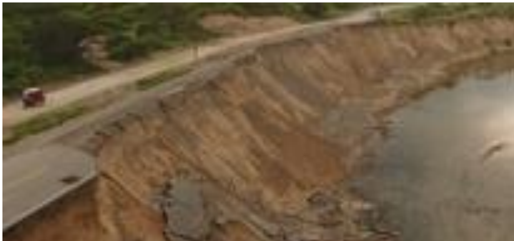
Km. 139+100- Km.139+300 – Tramo 5
