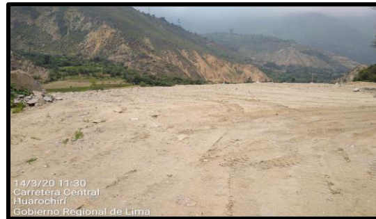
DME – Km. 068+000 SUB TRAMO 1
