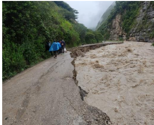
EV24-2022 ST03 KM129+500
