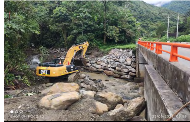
Enrocado Pte. Janneth – sector km 269+460
