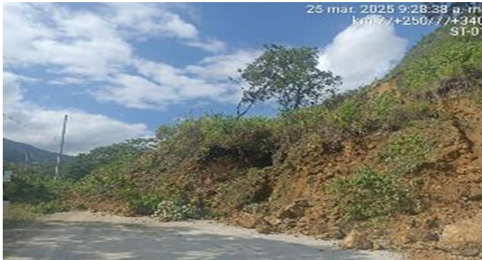
EV024-2025-ST01 km 77+250 – km 77+340
