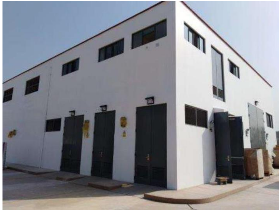
Fachada Principal SEAT terminada
