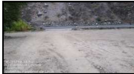
DME – Km. 068+000 SUB TRAMO 1
