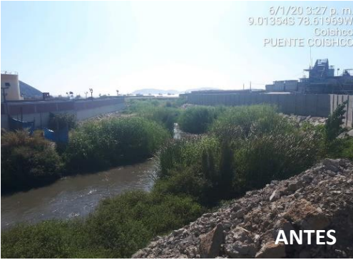
Puente Coishco - Km 443+720
