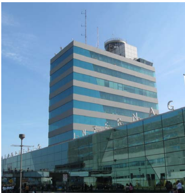
Vista exterior Torre central
